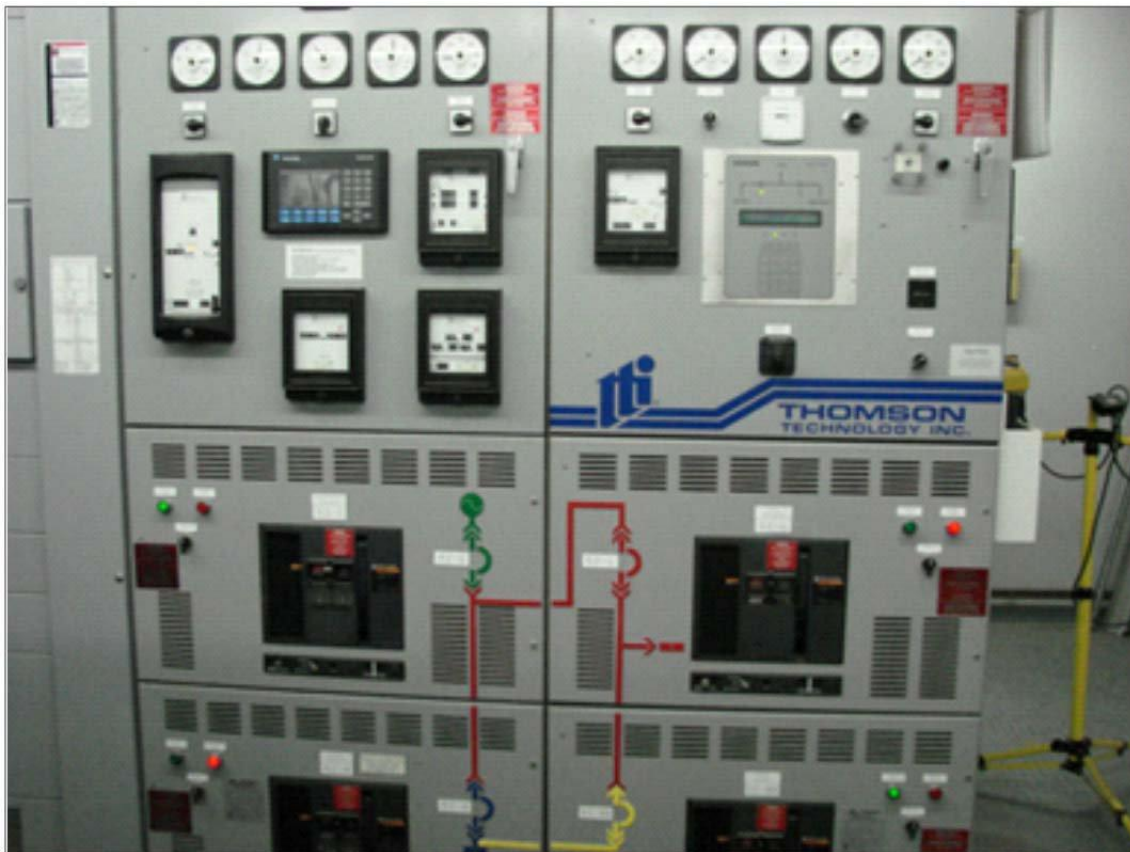
Figure 3-8. Transfer panel (source: Toronto International Airport)
