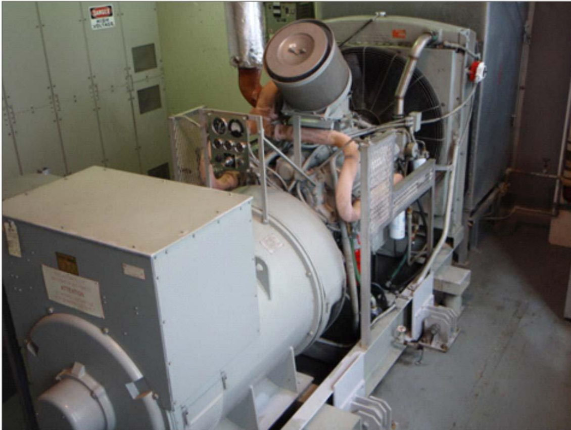
Figure 3-7. Diesel-electric generator set (source: Toronto International Airport)
